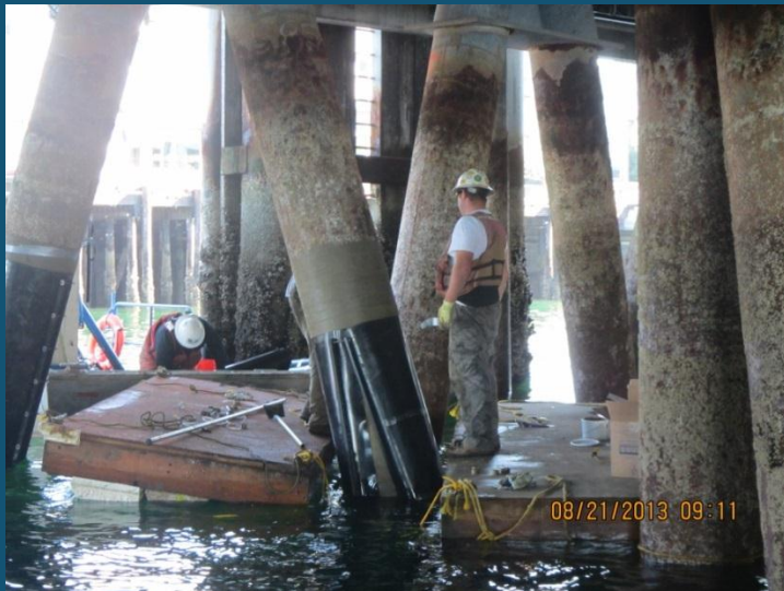
Before Beneficial Occupancy
